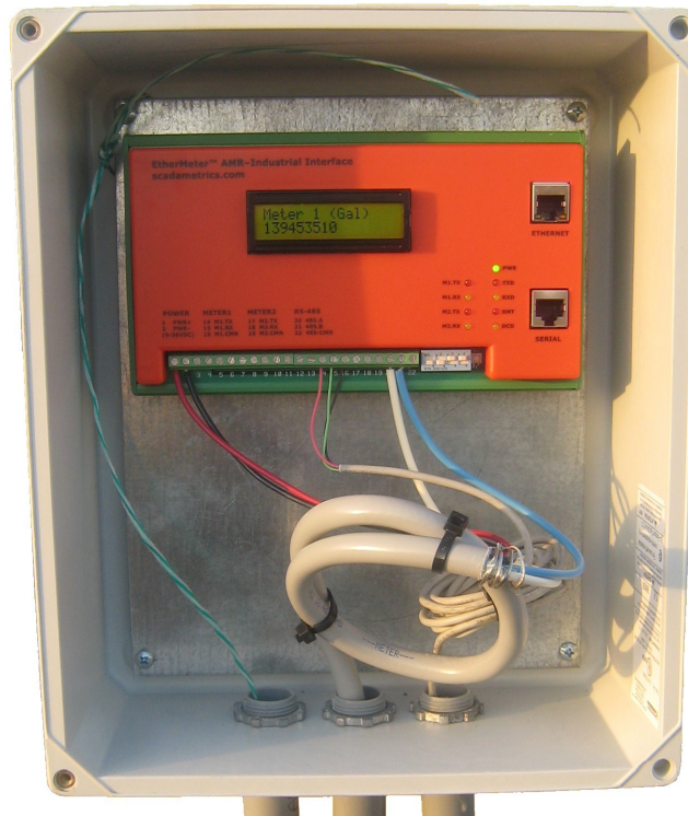
An Installed EtherMeter® AMR-Industrial Interface
