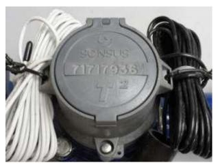
**Sensus Omni Register.** The Pulse Cable (L) has a GRAY jacket, and the Encoder Cable (R) has a BLACK jacket. The Encoder Cable is terminated with a touch-read pad, which should be cut/removed in order to expose the inner three conductors, which are color-coded RED, GREEN, BLACK.
