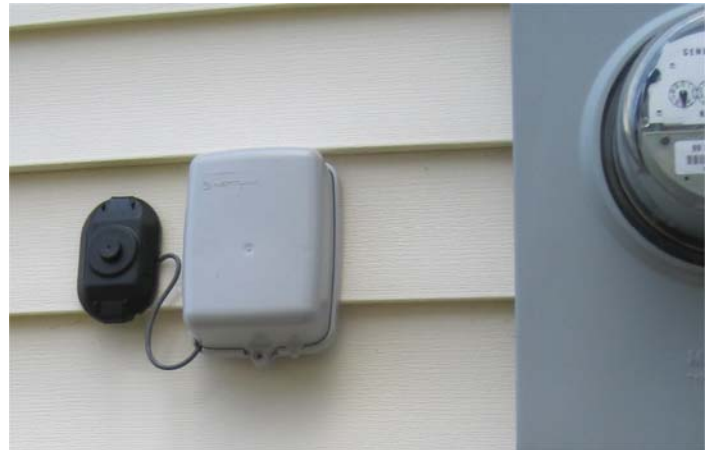
An Outdoor, Wall-Mounted Touch-Read Pad Can Now Co-Exist With An AMI Radio Endpoint.
